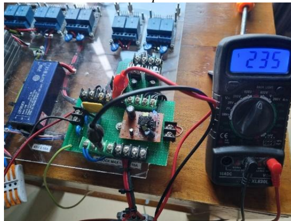
Figure 8. Testing power delivery
